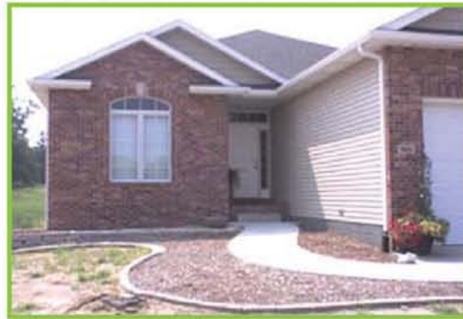
House built without LOW-E
