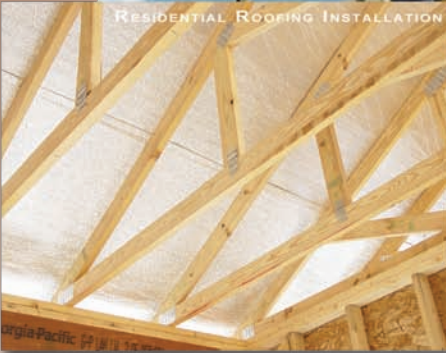
RESIDENTIAL ROOFING INSTALLATION
