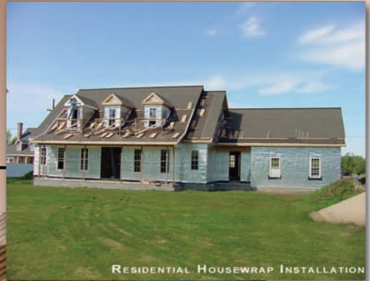
RESIDENTIAL HOUSEWRAP INSTALLATION
